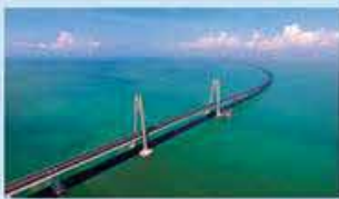
Hong Kong - Zhuhai - Macau Bridge
