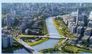
Western Bridge (The Loop Project)
